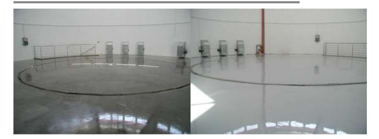
Resimac floor coatings are a range of solvent free epoxy resin based systems ideal for resurfacing and rebuilding concrete surfaces. Our range of materials can give a wear resistant and chemical protective finish to concrete surfaces in many industrial environments.
