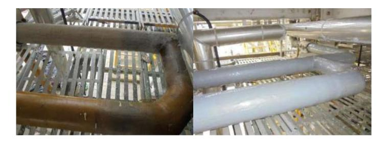
Resimac Liquid Insulation Composite coatings are based on a combination of innovative fillers bound in a 100% solids epoxy resin.
